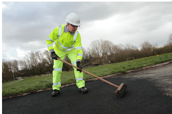
S106 monies secured for highways and infrastructure improvements
